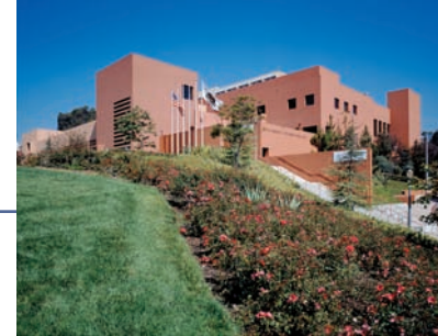
Bradley International Hall
