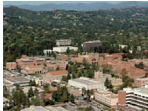
View of campus facing northwest
